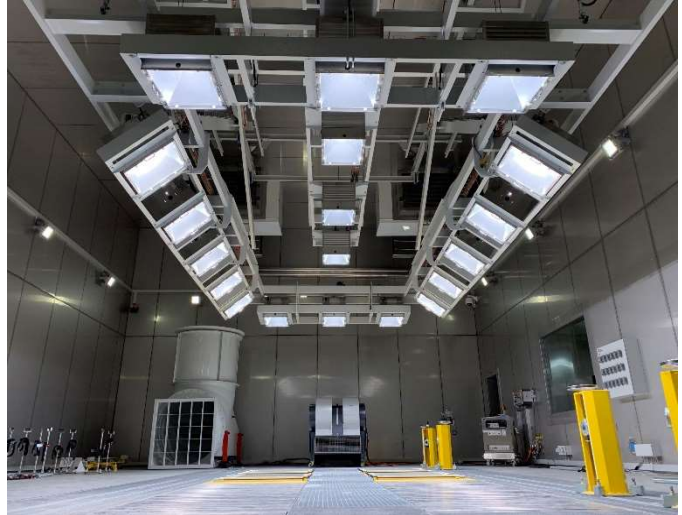
Figure 3: Drive-in chamber with 19x SolarConstant MHG 4000; inclined side frames.
