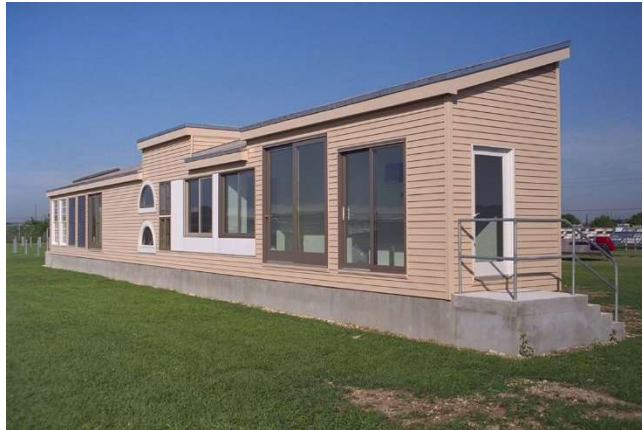
Figure 3. Test house at Atlas South Florida Test Service for exposure of window sealants in end-use.
